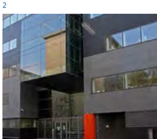
1 First building in Austria to be awarded a Green Building Certificate Johnson Controls Metasys® Building Automation System helps UNIQA Towers in Vienna achieve a Green Building Certificate for energy efficiency.
